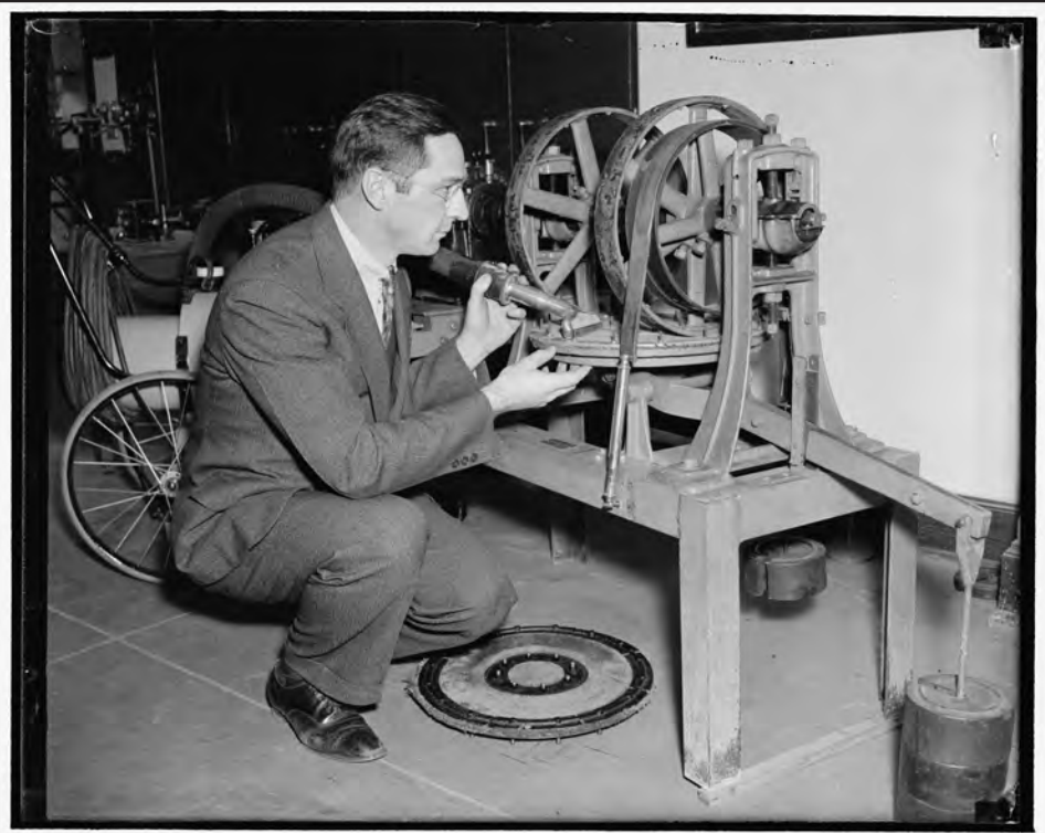
How much wear will your carpet stand? A machine that produces the bending, slipping, twisting, and compression of the pile that takes place when a carpet is walked upon, has been developed by the National Bureau of Standards to test the durability of carpets. H.F. Schiefer, physicist at the Bureau, is shown in the photograph, 3/19/38, Courtesy Library of Congress, Photo by Harris & Ewing.
