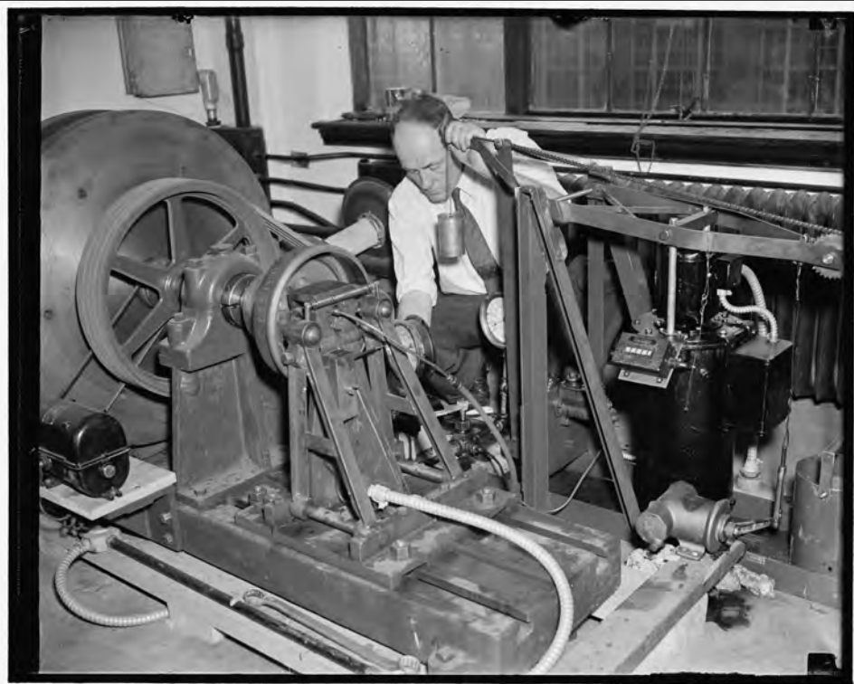
New machine to test brake linings designed by Bureau of Standards. A new machine, both in design and operations, has been installed at the National Bureau of Standards for the testing of brake linings. The machine permits the study of brake linings under conditions closely approaching those of actual service and yet which can be accurately controlled. It will make less difficult the complex job of revising the Federal Government's specification for auto brake linings. Wil. Holt of the Bureau is shown in the photograph, 3/16/38, Courtesy Library of Congress, Photo by Harris & Ewing.
